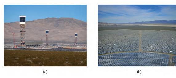
Figure 5.10 (a) The Ivanpah solar thermal plant uses 170,000 mirrors to concentrate sunlight on water-filled towers. (b) It covers 4000 acres of public land near the Mojave Desert and the California-Nevada border. (credit a: modification of work by Craig Dietrich; credit b: modification of work by "USFWS Pacific Southwest Region"/Flickr)
