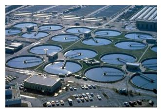
Figure 15.6 Wastewater treatment facilities, such as this one, remove contaminants from wastewater before the water is released back into the natural environment. (credit: "eutrophication&hypoxia"/Wikimedia Commons)
